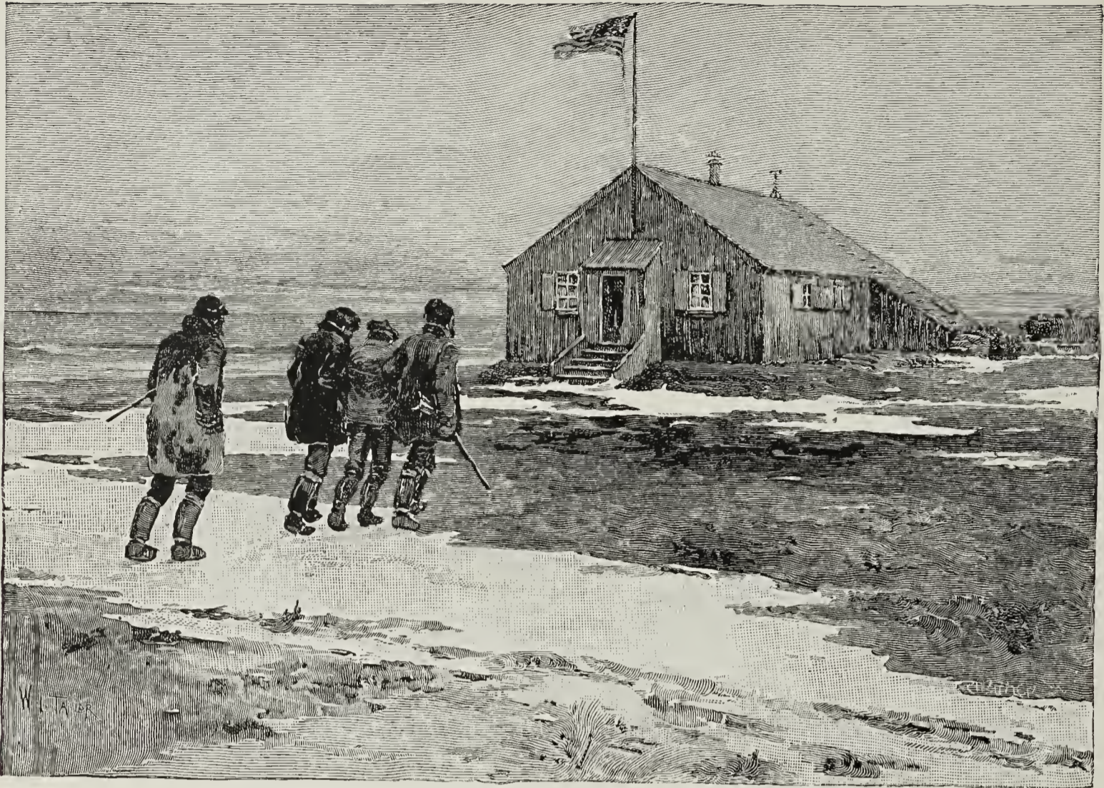
Refuge Station, Point Barrow, Alaska. (See page 1281.) (Courtesy of Scribner's Magazine.)
